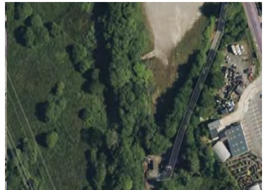
Figure 11-3 – Possible Underbridge Obstruction – BA-01-02
