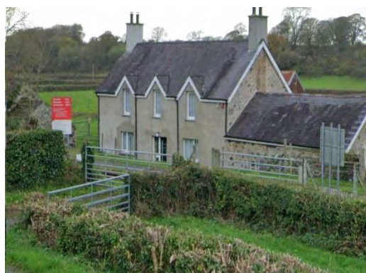
Figure 8-19 – Access track crosses alignment Obstruction - CD-02-04
