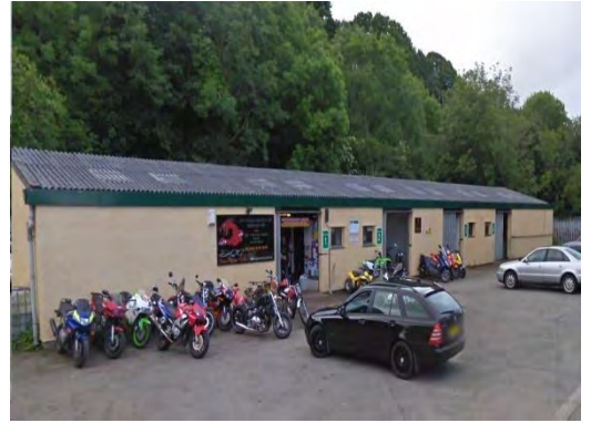
Figure 7-27 – Commercial premises adjacent to Port Dinorwic Station. Obstruction BC-06-04
