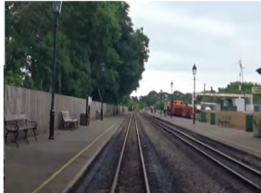
Figure 8-32 – Dinas Station Platforms Obstruction - CD-04-04
