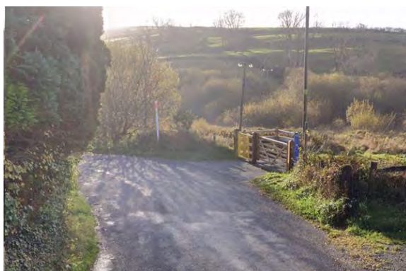
Figure 10-19 – Local Road Crossing near former station Obstruction Number – PB-06-02
