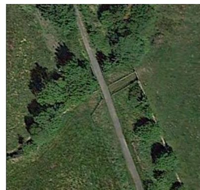
Figure 10-20 – Access Track Crossing Obstruction Number –PB-06-03
