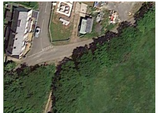
Figure 11-24 – Road crosses alignment Obstruction – BA-05-04
