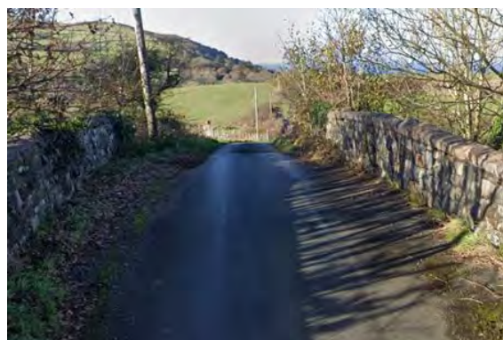
Figure 10-10 – Stone overbridge carrying local road Obstruction Number – PB-03-01
