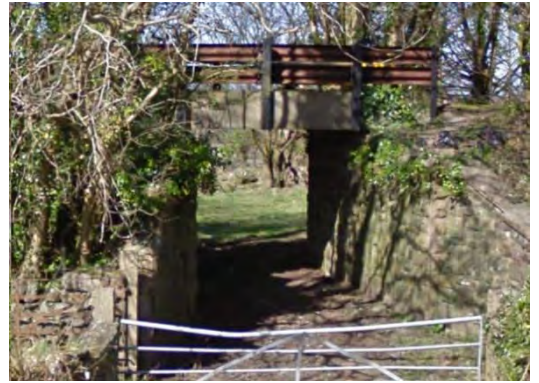
Figure 9-14 – Underbridge over access road Obstruction Number – DP-03-02
