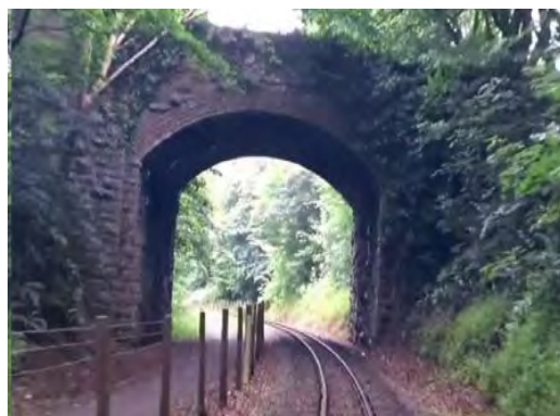
Figure 8-30 – Overbridge crosses alignment Obstruction - CD-04-02
