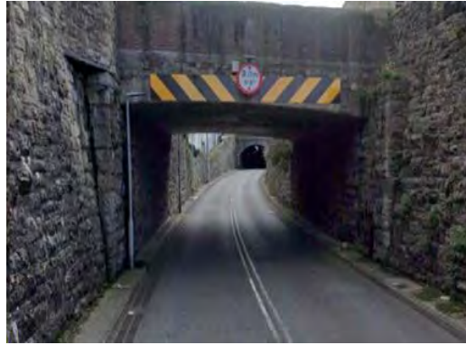
Figure 7-56 – Overbridge crosses alignment Obstruction BC-11-07
