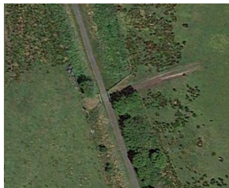
Figure 10-16 – Access Track Crossing Obstruction Number – PB-05-04
