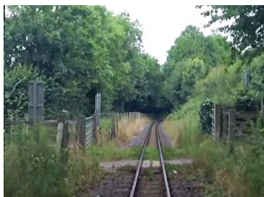
Figure 8-21 – Access track crosses alignment Obstruction - CD-02-06
