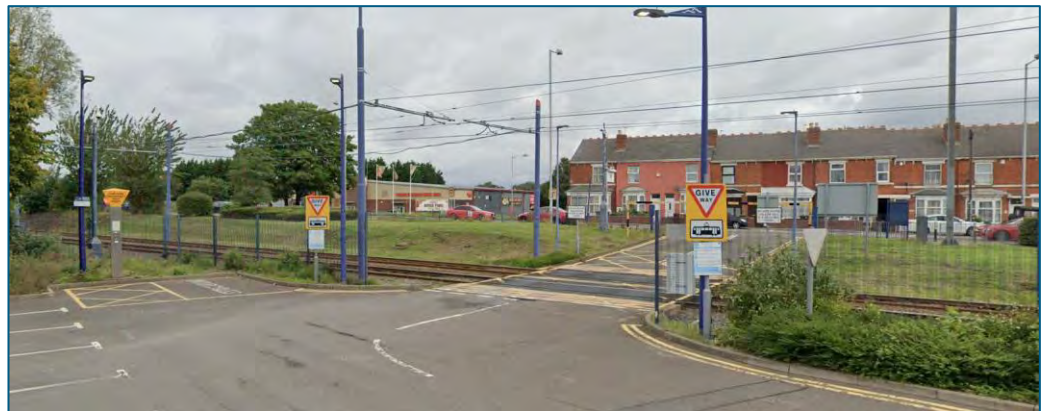
Figure 5-3 – Example Give Way junction on segregated Tram Lines – Priestfield Tram Stop Car Park on West Midlands Metro
