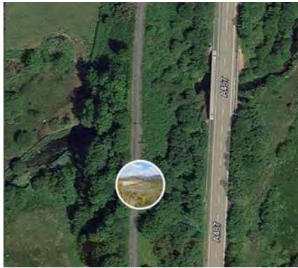
Figure 10-2 – Underbridge across Afon Llyfni Obstruction Number – PB-01-01
