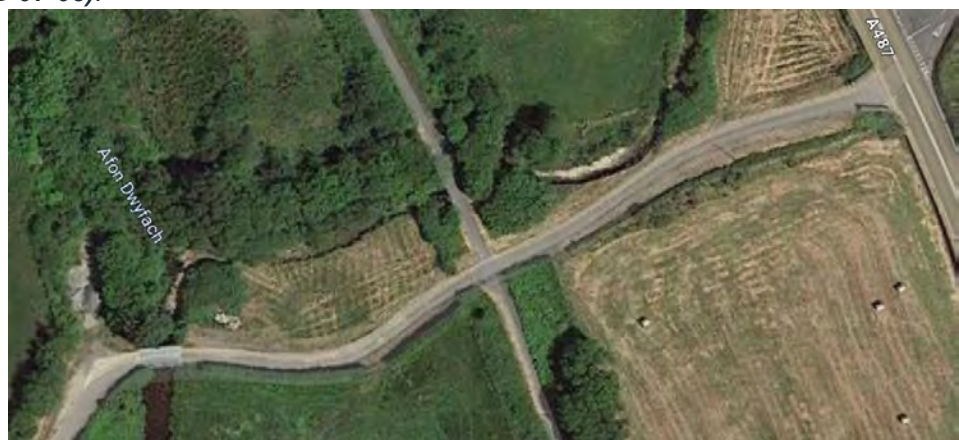
Figure 10-25 – Underbridge over tributary to Afon Dwyfach and Access Track crosses alignment Obstruction Number – PB-07-02 and PB-07-03
