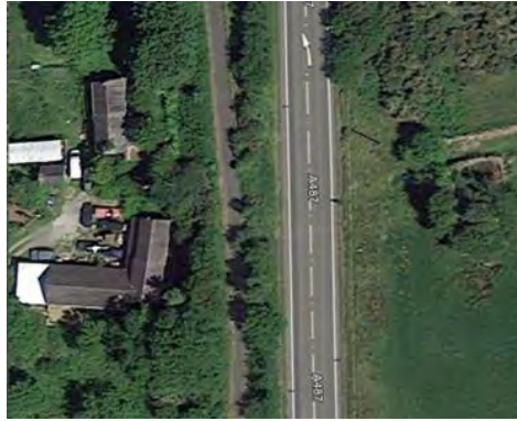
Figure 10-7 – Possible underbridge / culvert Obstruction Number – PB-02-02
