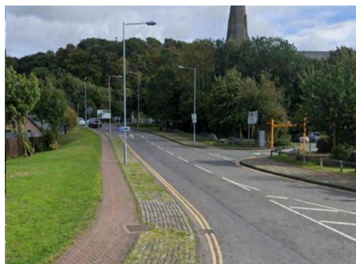
Figure 7-53 – Balaclava Road crosses alignment Obstruction BC-11-04
