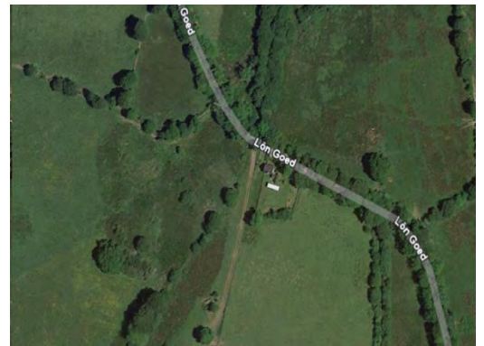
Figure 11-19 – Access track crosses alignment Obstruction – BA-04-02
