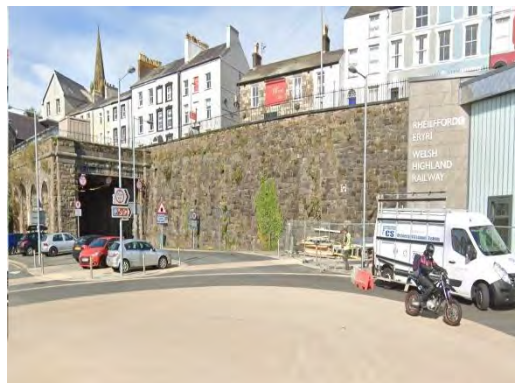
Figure 8-2 – South Portal of Caernarfon Tunnel
