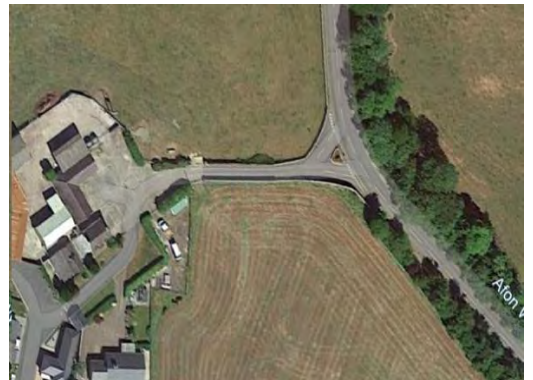
Figure 11-40 – Access Road crosses alignment Obstruction – BA-07-07
