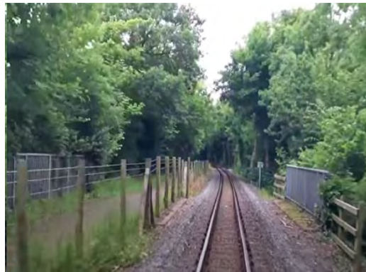
Figure 8-28 – Underbridge over access track Obstruction - CD-03-05
