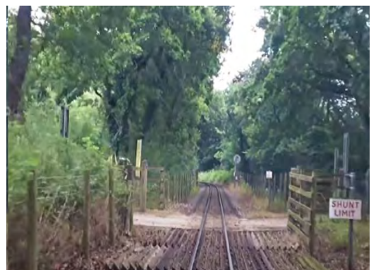
Figure 8-31 – Access track crosses alignment Obstruction - CD-04-03
