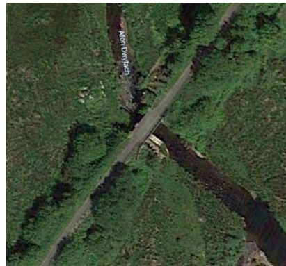
Figure 10-26 – Underbridge over Afon Dwyfach Obstruction Number – PB-07-04
