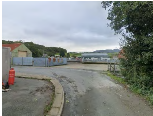
Figure 10-31 – Commercial business constructed on alignment Obstruction Number – PB-08-04
