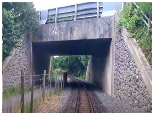
Figure 8-12 – St Helens Road overbridge crosses alignment Obstruction - CD-01-05
