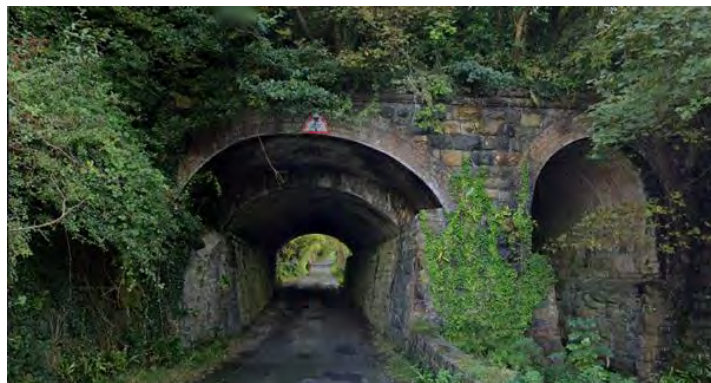
Figure 10-3 – Underbridge across Afon Crychddwr and local road Obstruction Number – PB-01-02
