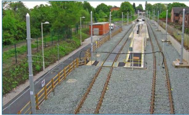
Figure 9-27 – View of St. Werburgh's Road Tram Stop on Manchester Metrolink, showing typical station pedestrian crossing point at end of platforms 19
