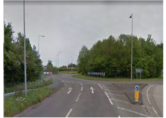
Figure 7-39 – Plas Menai Roundabout intersects alignment Obstruction BC-08-03
