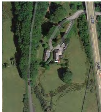
Figure 10-4 – Possible Underbridge Obstruction Number – PB-01-03
