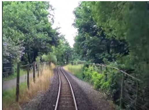
Figure 8-10 – Potential underbridge Obstruction - CD-01-04
