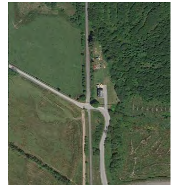
Figure 10-11 – Local Access Road near Cefn Graianog Obstruction Number – PB-04-01
