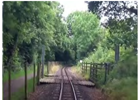
Figure 8-29 – Access track across alignment Obstruction - CD-04-01
