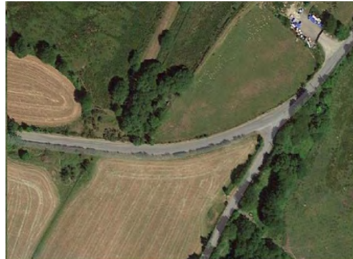
Figure 11-7 – Road crosses alignment Obstruction - BA-02-01
