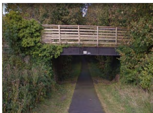
Figure 7-36 – Overbridge crosses alignment Obstruction BC-07-04
