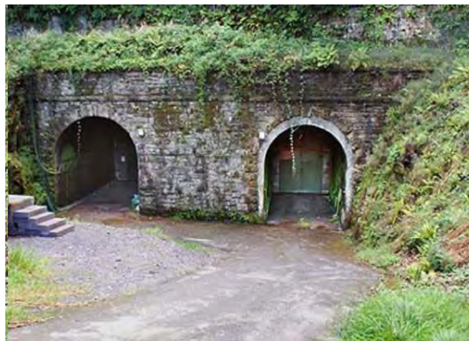
Figure 7-13 – Vaynol Tunnel Obstruction Number - BC-04-03
