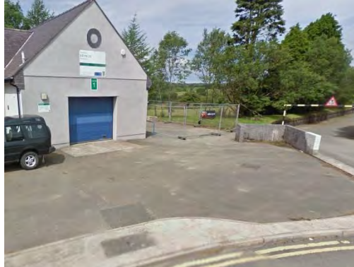
Figure 10-30 – Commercial business constructed on alignment Obstruction Number – PB-08-03
