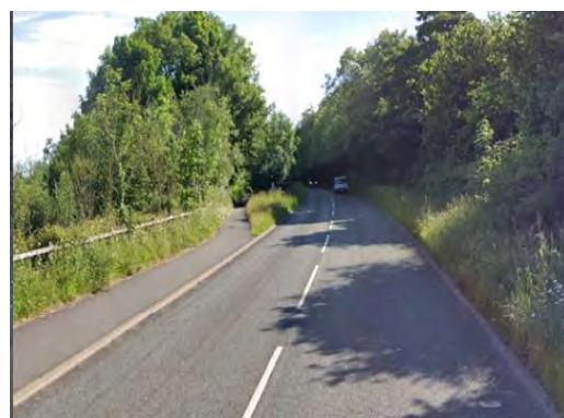
Figure 7-37 – Caernarfon Road intersects alignment Obstruction BC-08-01
