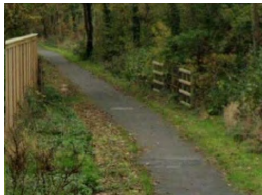
Figure 9-4 – Afon Rhyd underbridge Obstruction Number – DP-01-03
