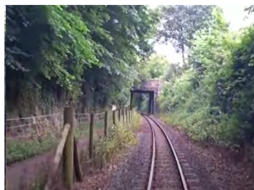
Figure 8-17 – Retaining walls along alignment Obstruction - CD-02-01
