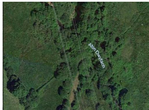
Figure 11-4 – Possible Underbridge Obstruction – BA-01-03
