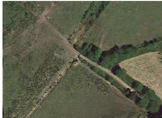
Figure 11-28 – Access track crosses alignment Obstruction - BA-06-02
