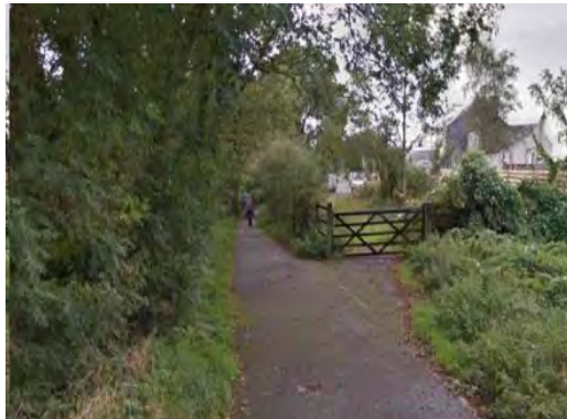
Figure 7-48 – Access track along alignment Obstruction BC-10-02
