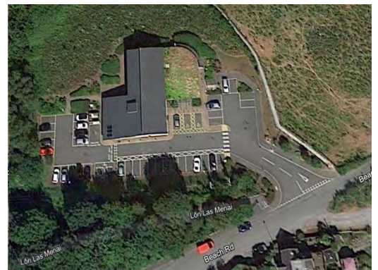
Figure 7-34 – New development adjacent to the alignment
