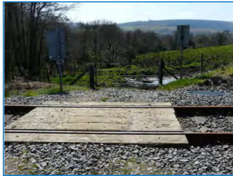
Figure 5-5 – Example User Worked Crossing (near Aberdare, South Wales), showing signage and gates
