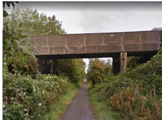
Figure 7-44 – Overbridge crosses alignment Obstruction BC-09-02
