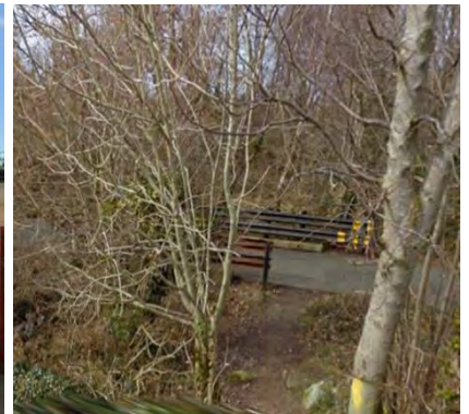
Figure 9-16 – Culvert under alignment Obstruction Number – DP-03-04
