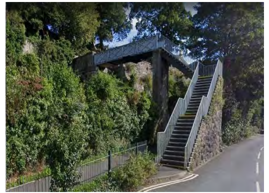
Figure 8-9 – Footbridge crossing alignment Obstruction - CD-01-03
