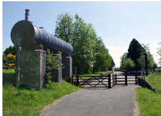
Figure 10-28 – View of Water Tank towards car park Part of Obstruction Number – PB-08-03 21
