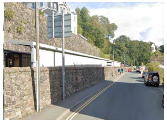
Figure 8-7 – Welsh Highland Railway Station Platform - Obstruction - CD-01-01
