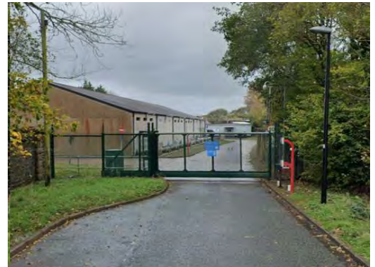
Figure 7-8 – Waterworks on alignment Obstruction Number – BC-03-04
