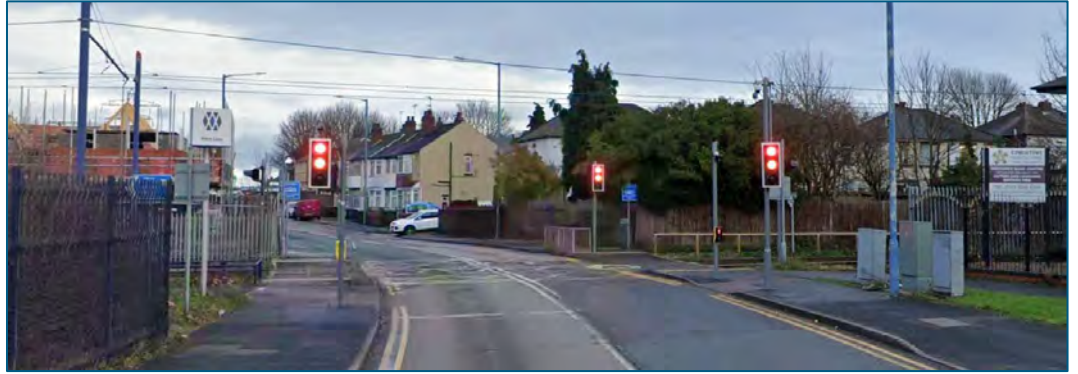
Figure 5-4 – Example Traffic Light Controlled junction on segregated Tram Lines – New Swan Lane on West Midland Metro
