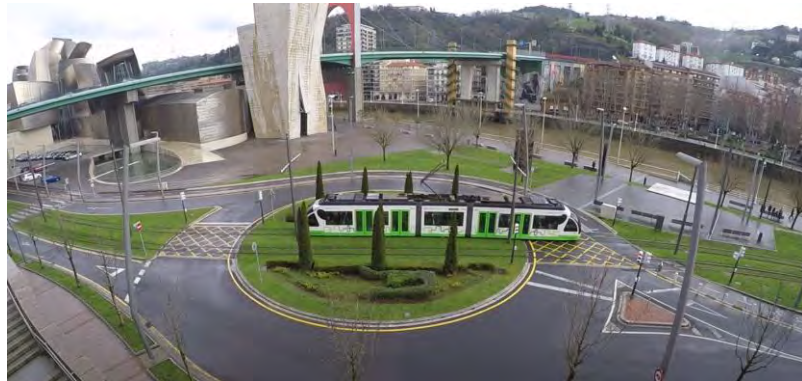
Figure 9-7 – Roundabout with tram lines through centre and traffic light controls (Bilbao, Spain)
