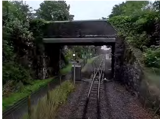
Figure 9-2 – Ty'n Llan road overbridge Obstruction Number – DP-01-01
