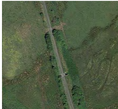
Figure 10-15 – Access Track and Underbridge Obstruction Number – PB-05-03
