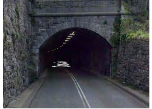
Figure 7-57 – Tunnel along alignment Obstruction BC-11-08
