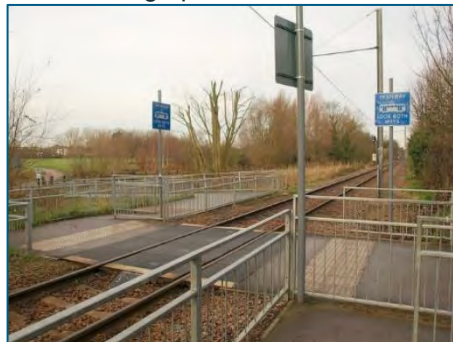
Figure 5-6 – Example of passive pedestrian crossing (e.g. with no additional protection measures) across segregated Tram Lines – Morden Hall Park footpath crossing on London Tramlink 18
