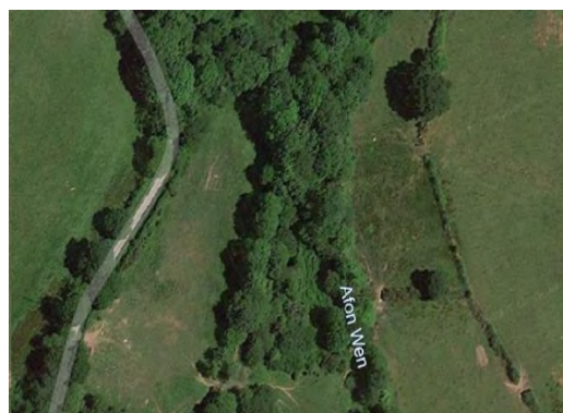
Figure 11-30 – Possible Underbridge Obstruction - BA-06-04
