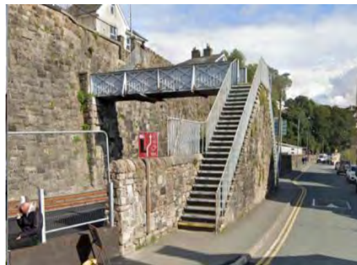
Figure 8-6 – Footbridge crossing alignment Obstruction - CD-01-02
