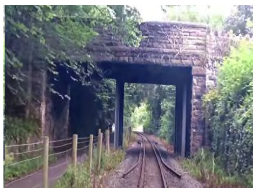
Figure 8-16 – Overbridge carrying Coed Helen Lane Obstruction - CD-01-08
