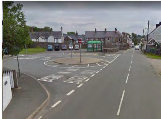
Figure 11-37 – B4354 crosses alignment Obstruction - BA-07-04
