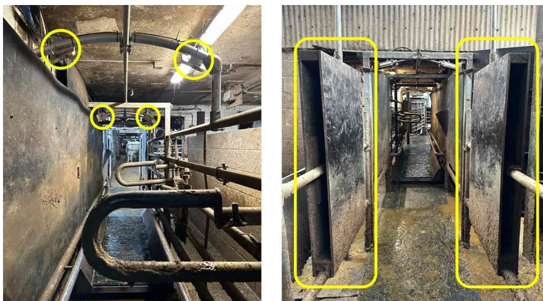
Figure 2.3. The four-antenna UHF static reader (left, antennas circled in yellow) and the HerdVision LF EID panels (right, within the yellow boxes) installed on the main parlour exit race. Cows exiting from the parlour pass the UHF antennas followed by the HerdVision system. The photograph on the left shows the cow's view when exiting, and the photo on the right is looking back up the race towards the rotary parlour.
