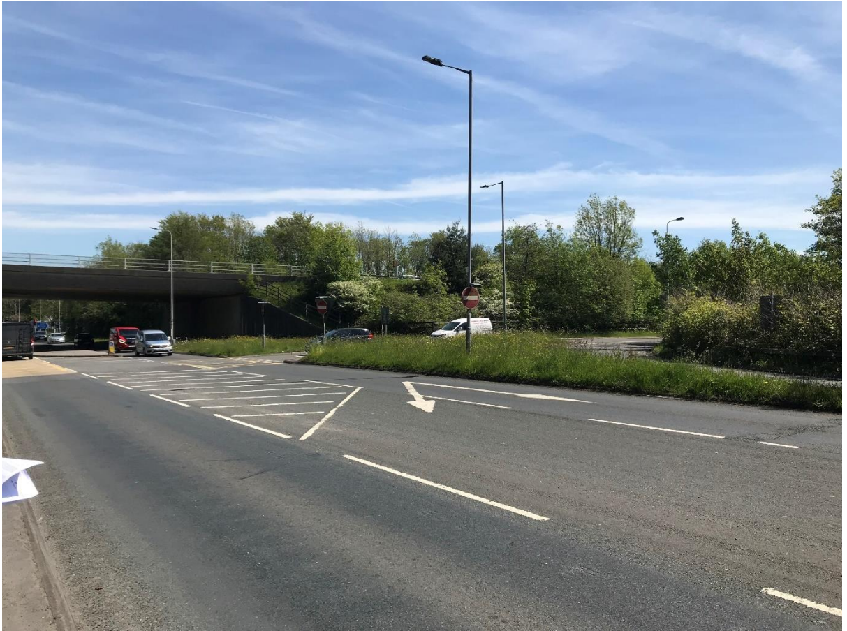
Figure 2-3 View of M4 J48 WB exit intersection with the A4138
