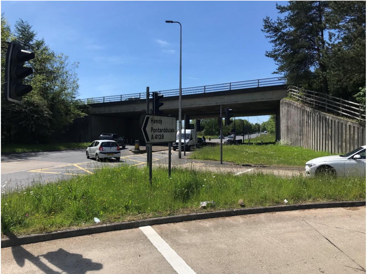
Figure 2-4 View of M4 J48 EB exit intersection with A4138
