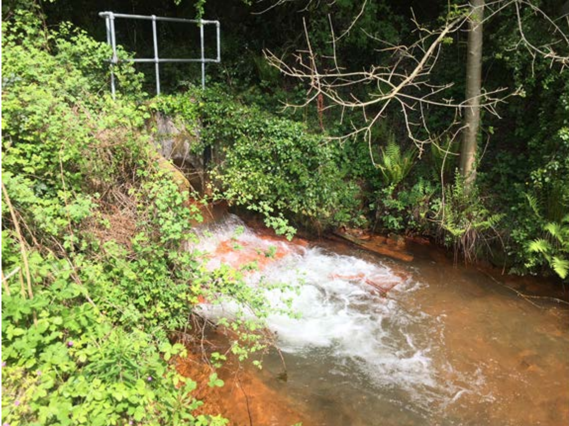
Figure 5.2: Abersychan discharge and Cwmsychan steam culvert discharge
