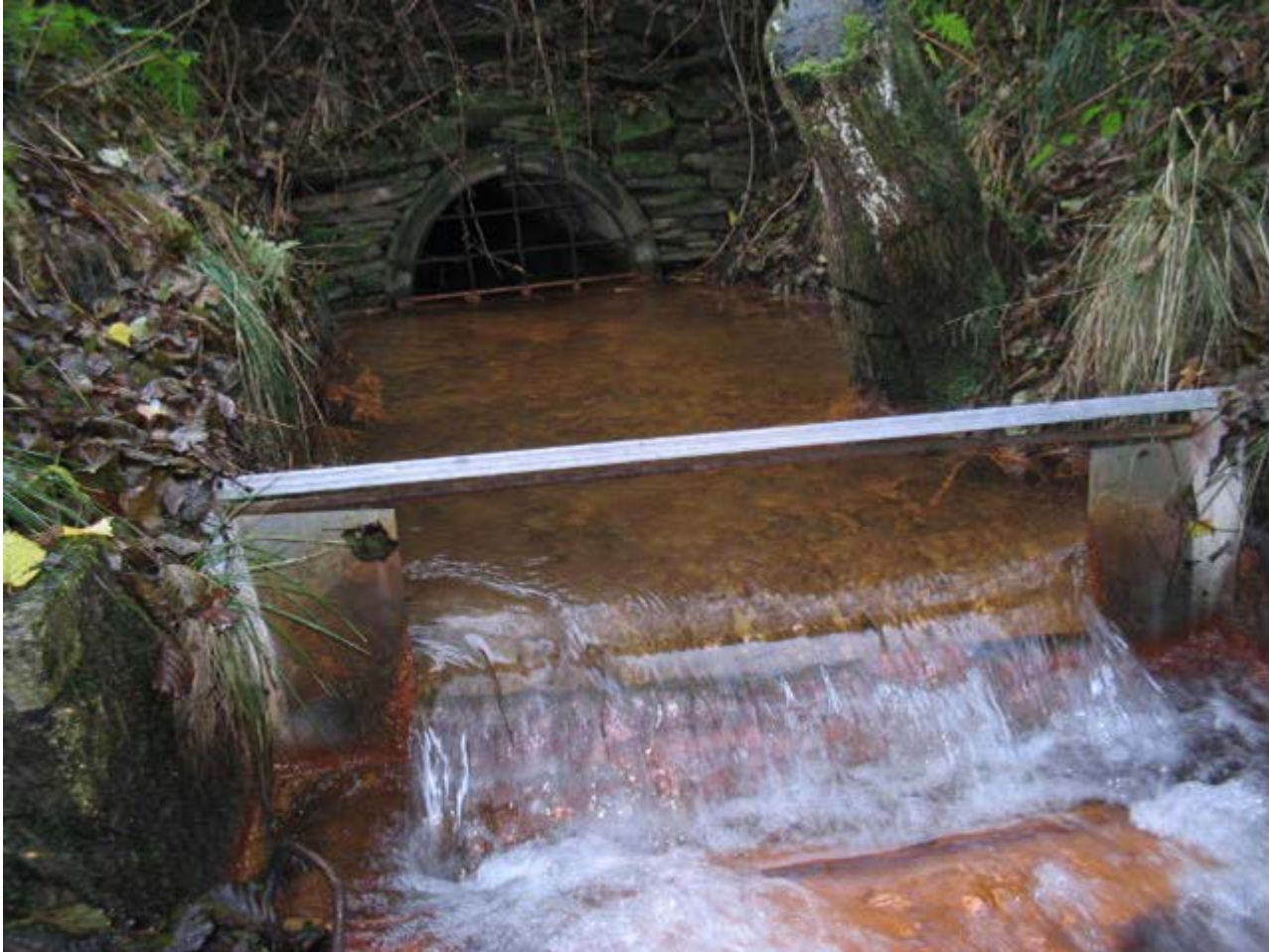
Figure 5.2: Photograph of Castle Shaft Discharge
