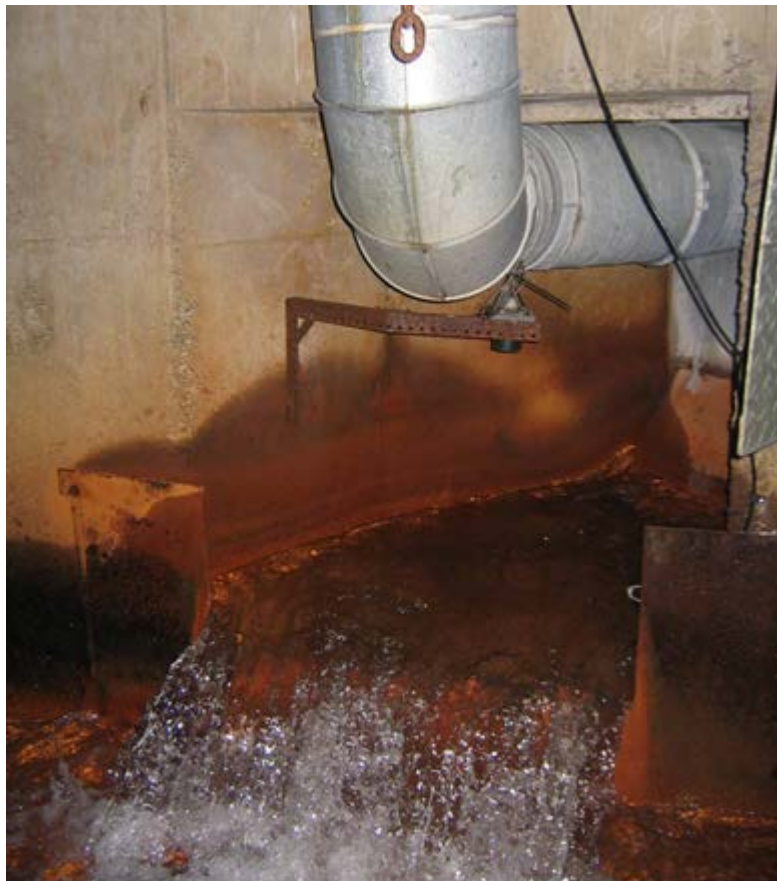
Figure 5.6: Pontlloctyn Bute Level discharge to river culvert
