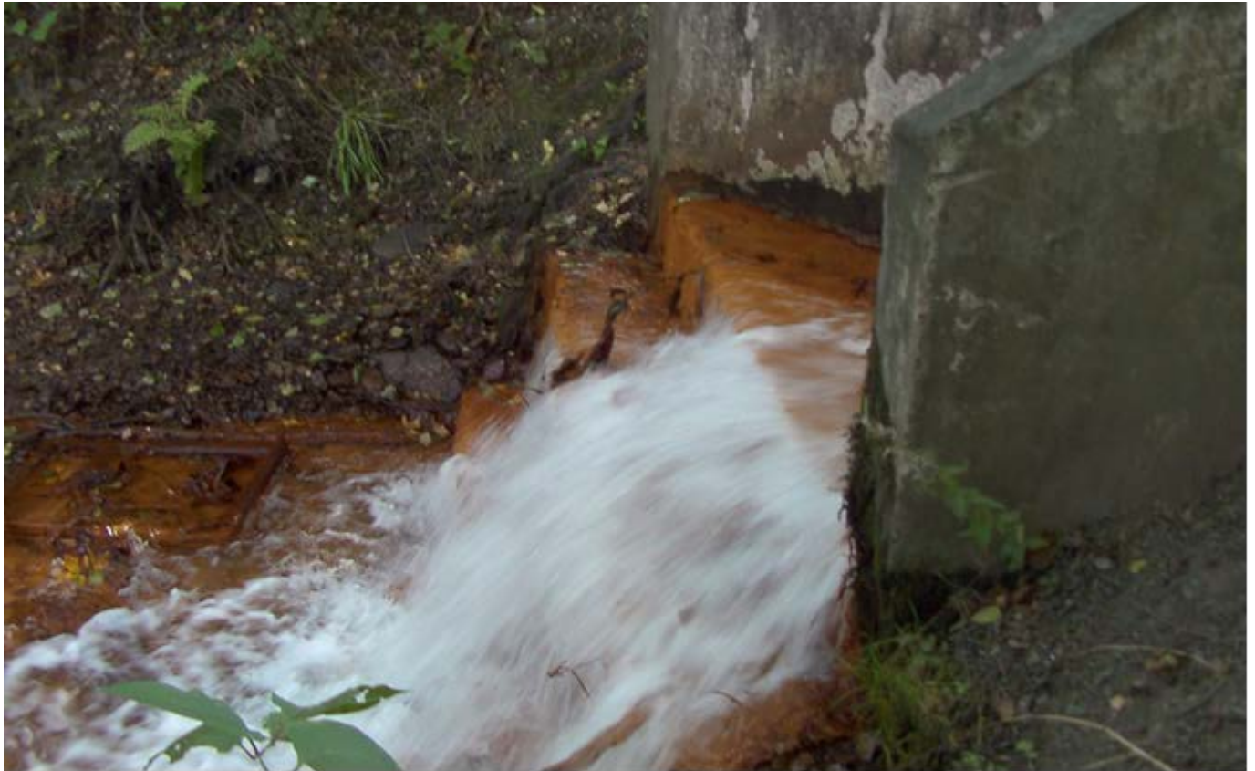
Figure 5.9: Tram Road Discharge
