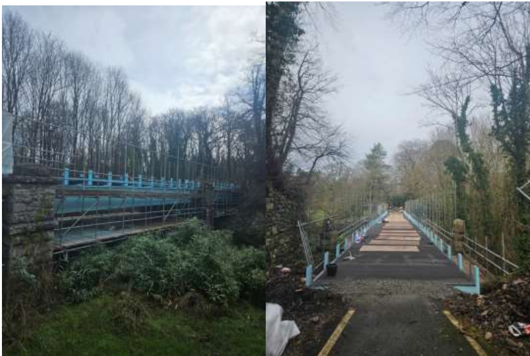
Route 82 - Lon Las Ogwen - New bridges installation
