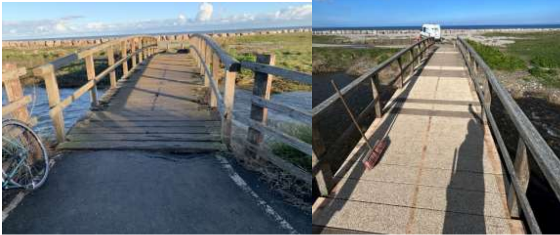
Dulas Bridge repairs - NCN 5, Conwy
