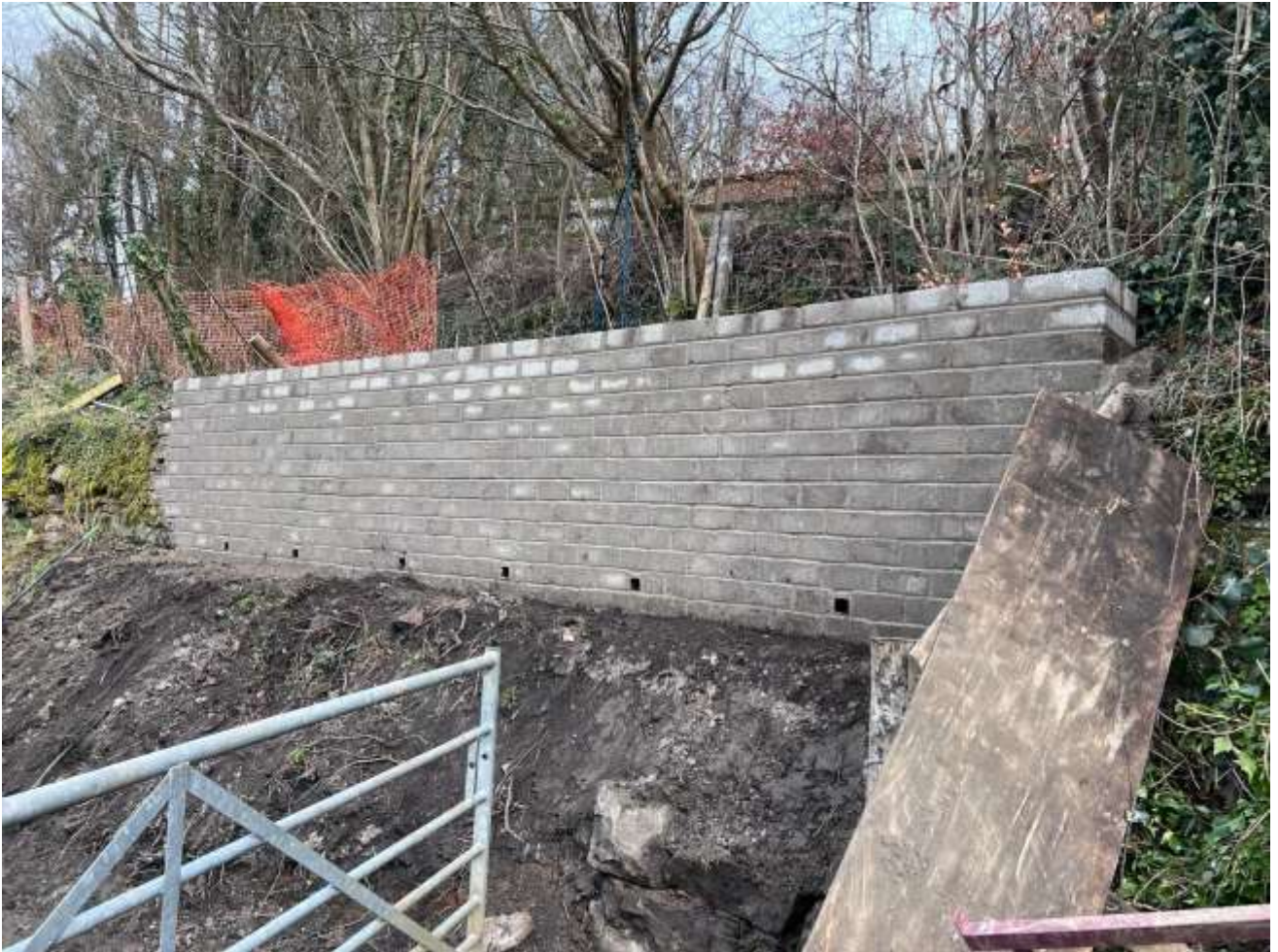
New retaining wall, Box cottage, Clydach Gorge
