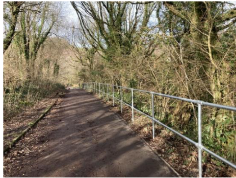
New fence at Hengoed
