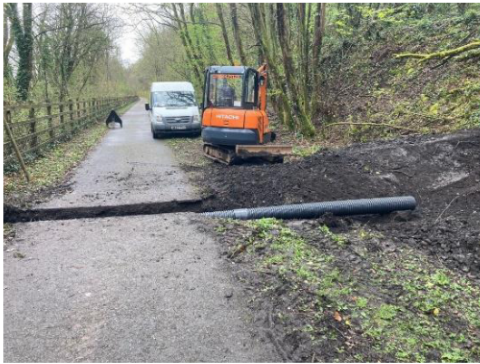
Drainage works at Treforest
