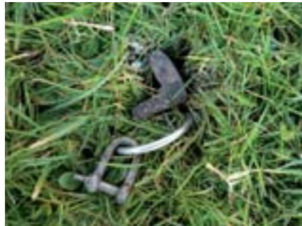
Angle iron anchor stake in position.
