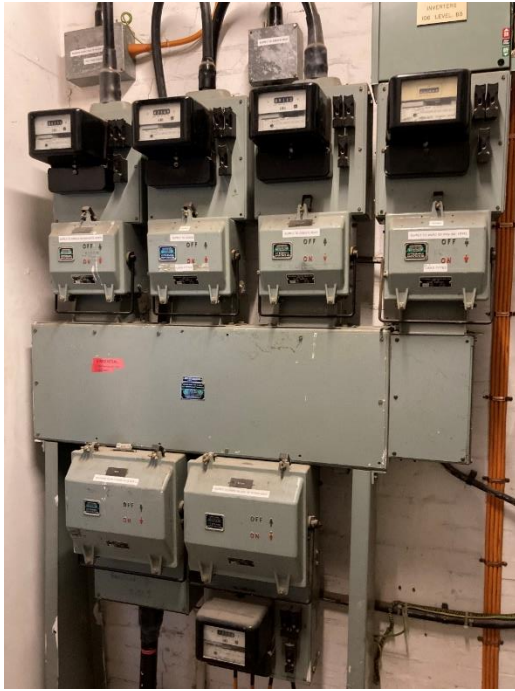
Typical LV main switch-room arrangement. Typical Ward Block riser main switchgear arrangement.
