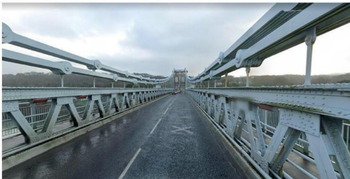
Figure 3 - View at deck level looking toward Bangor
