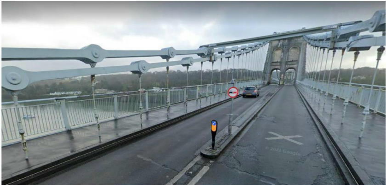
Figure 4: Anglesey Approach Span
