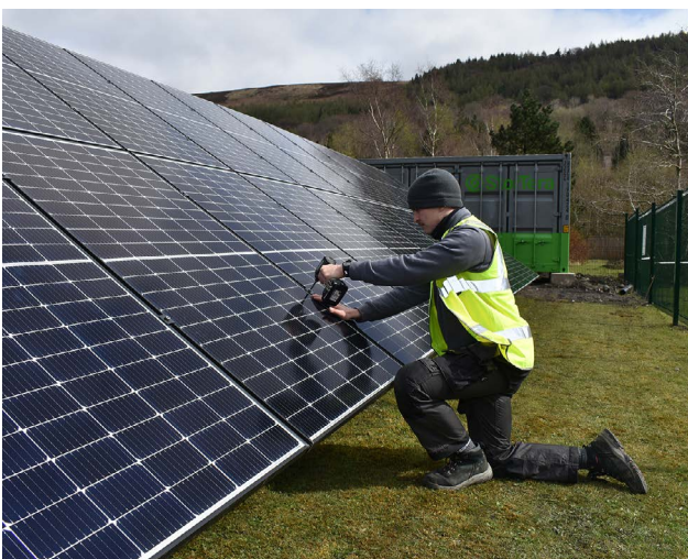
Solar panels being installed on site at Roseheyworth Business Park.
