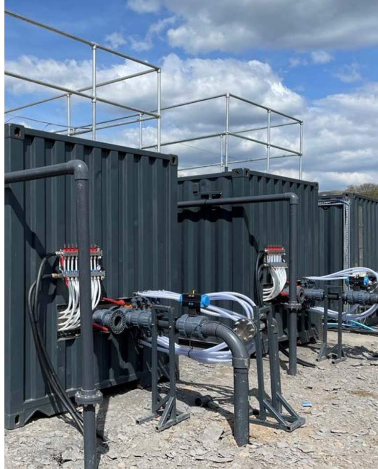
BioFactory anaerobic digester demonstrator at Coleg Llysfasi farm (WBRID Net Zero Farm Challenge).
