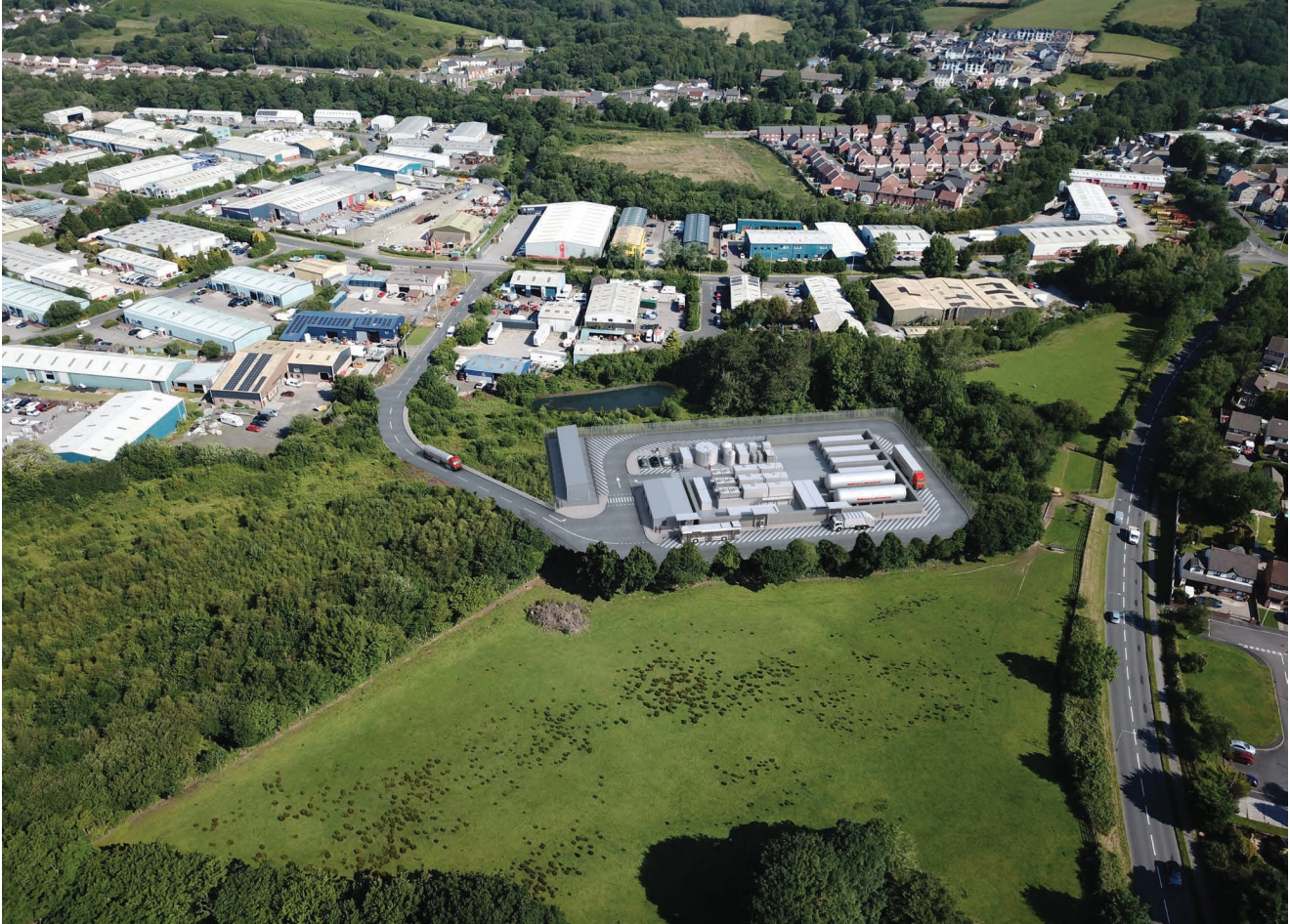
Aerial visualisation of proposed HyBont green hydrogen production facility at Brynmenyn, Bridgend.
