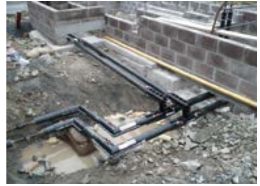
Connection branch pipes to customer properties Reproduced with permission of SHEaP
