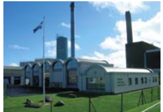
Peak load boiler station and thermal store Reproduced with permission of SHEaP
