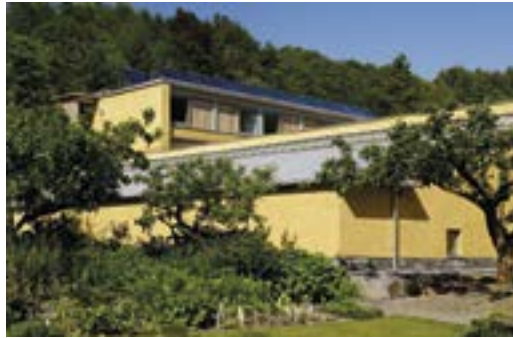
Biomass CHP unit installed at CAT Reproduced: Need approval from CAT, media@cat.org.uk
