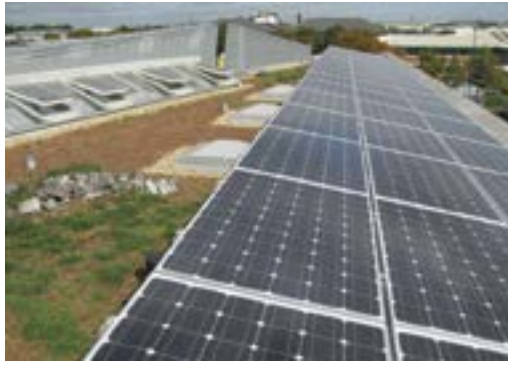
Large PV array and open roof windows Reproduced with permission of Stride Treglown
