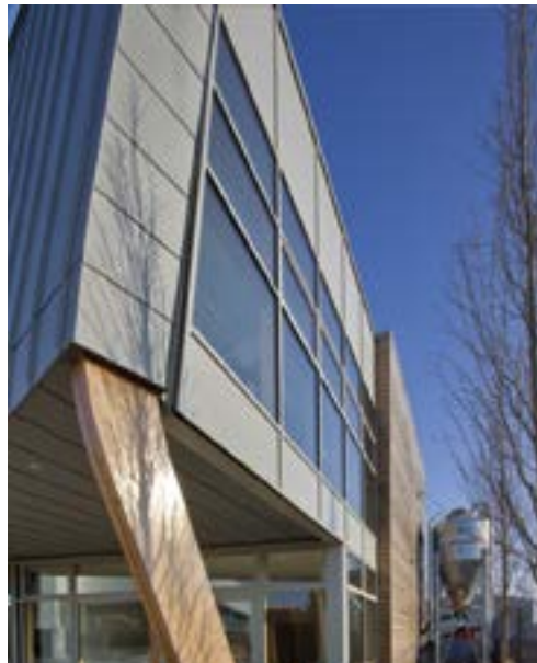
Timber and recycled Falzinc facades with biomass pellet hopper in background Reproduced with permission of Stride Treglown
