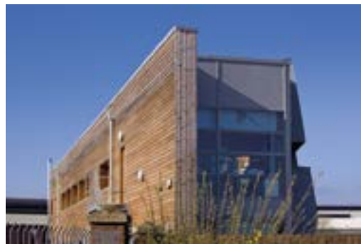
Solar PV array on southern facade Reproduced with permission of Stride Treglown
