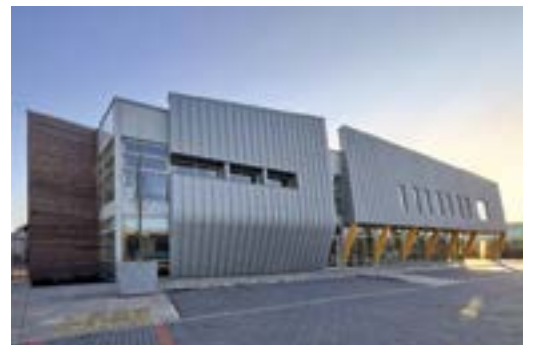
The new Treglown Court Office building Reproduced with permission of Stride Treglown
