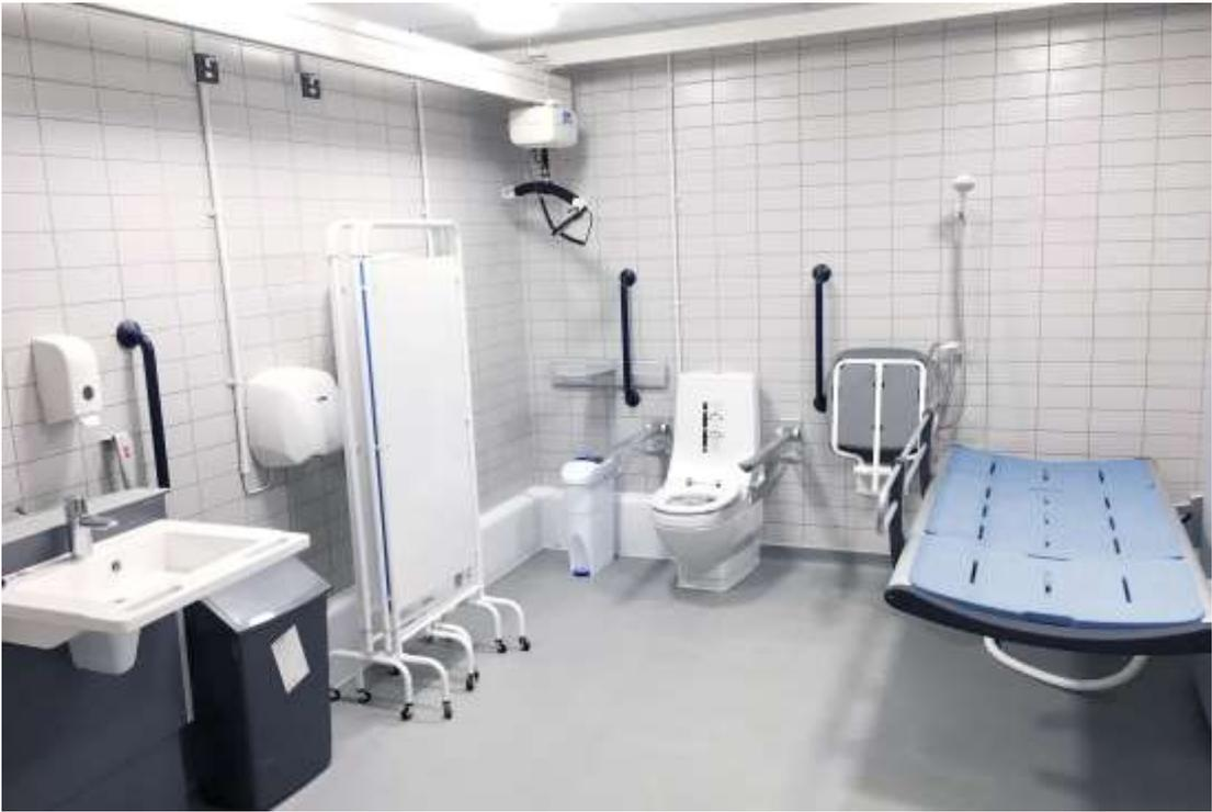
Figure 2 – Indicative CPT Layout and Equipment:
